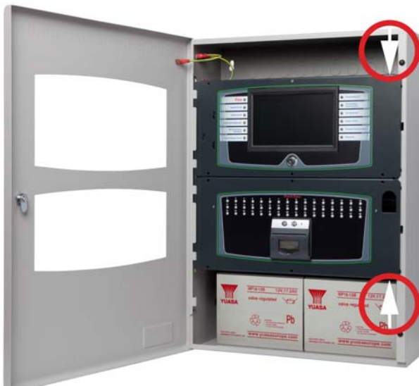
Figure 3-6 Opening the Fascia
