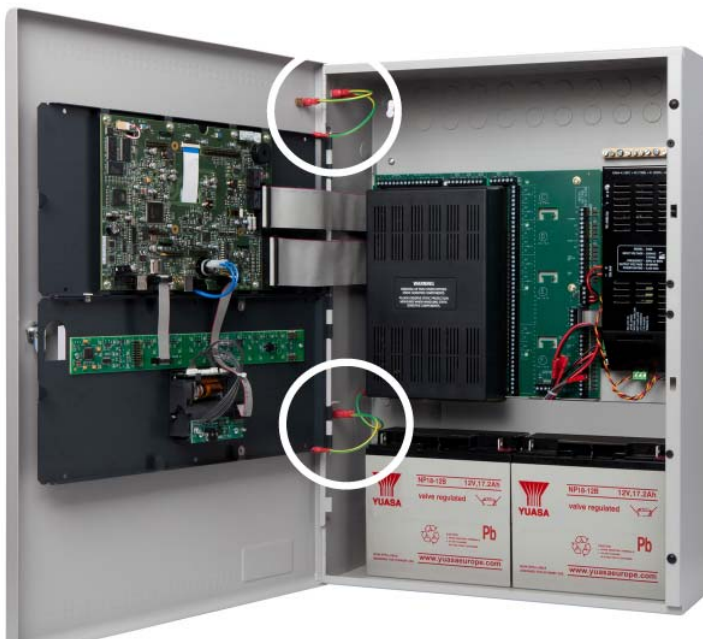
Figure 3-7 Removing Earth Bonding connections
